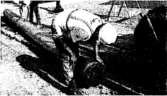
Touhy Avenue Water Main Replacement Niles, IL (Ciorba Group) Ongoing
