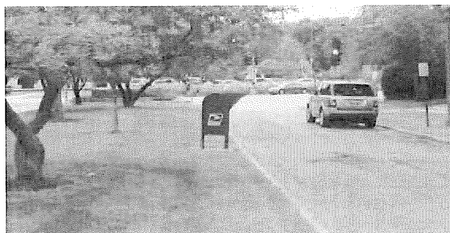
Kenilworth Water Interconnection Design The Villages of Kenilworth and Wilmette, IL (Stanley Consultants) 2015
